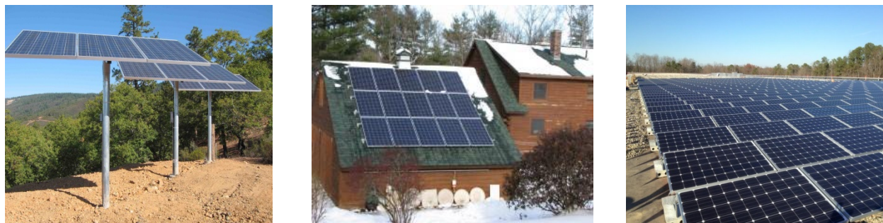
Figure 38 Ground-mounted system, Roof-mounted system and PV Farm
