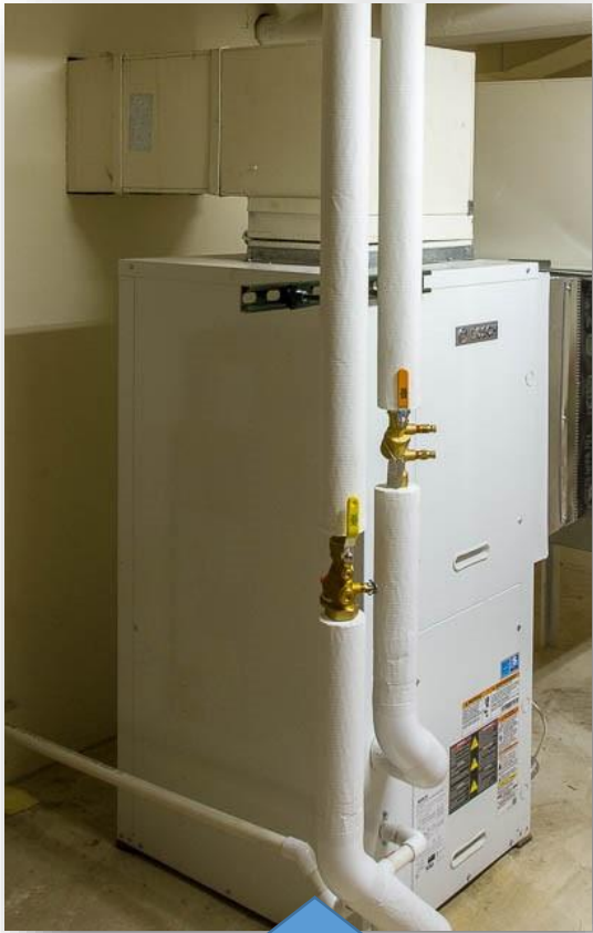
Vertical GHP (water-to-air GHP)
