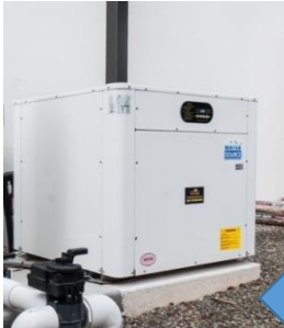
Horizontal; GHP (water-to-air GHP)
