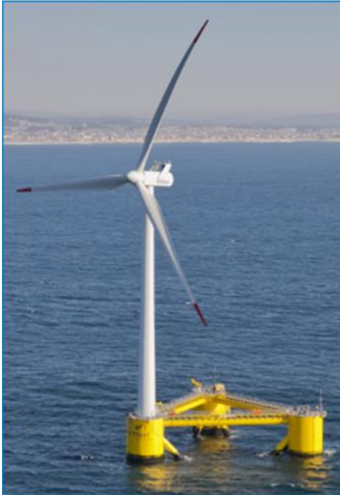
Principle Power 2.0-MW floating wind turbine in Portugal; 2011 WindFloat semisubmersible substructure. Photo by Walt Musial, NREL
