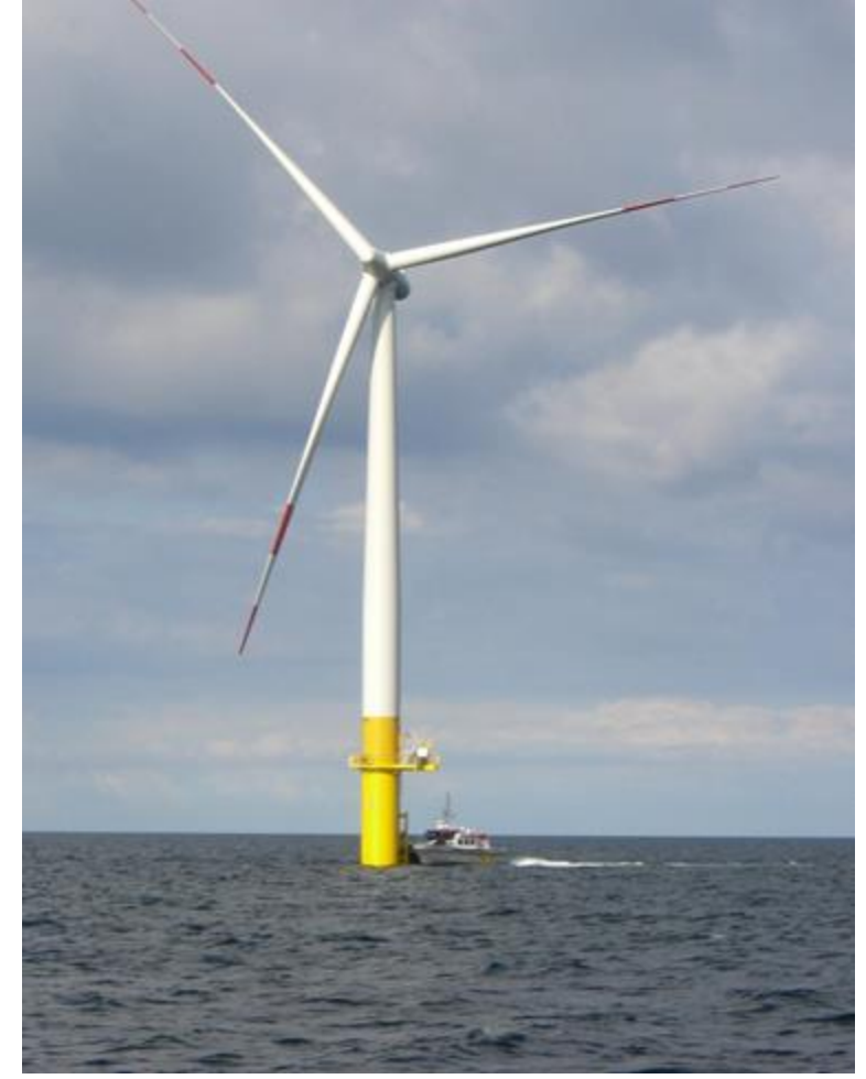
Baltic-1 2.3-MW Siemens fixed-bottom wind turbine in Germany; 2010 monopile substructure. Photo by Walt Musial
