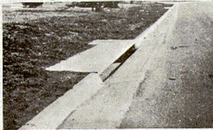
A - Curb-opening Inlet.
