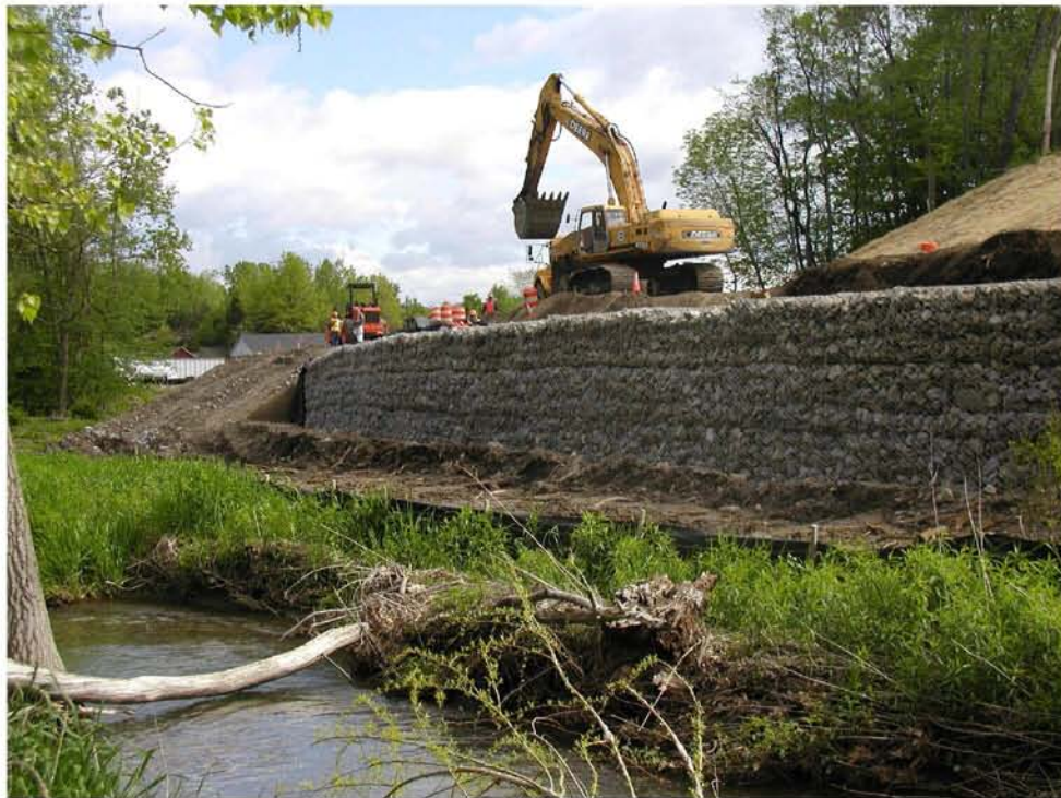
FIG. 27 GABION WALL CONSTRUCTION
