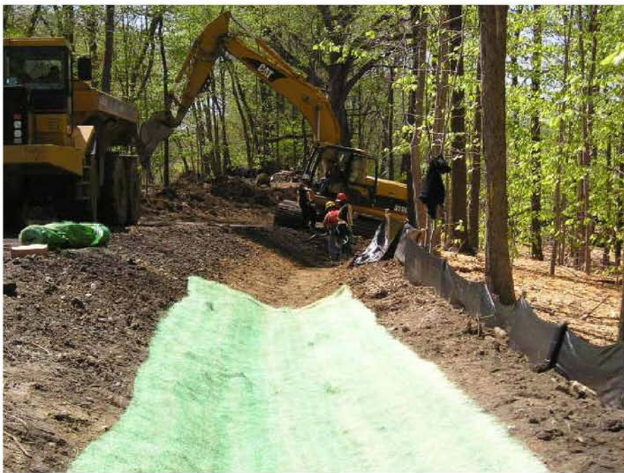
FIG. 19 INSTALLATION OF EROSION CONTROL MAT FOR STABILIZATION OF GRASS LINED SWALE
