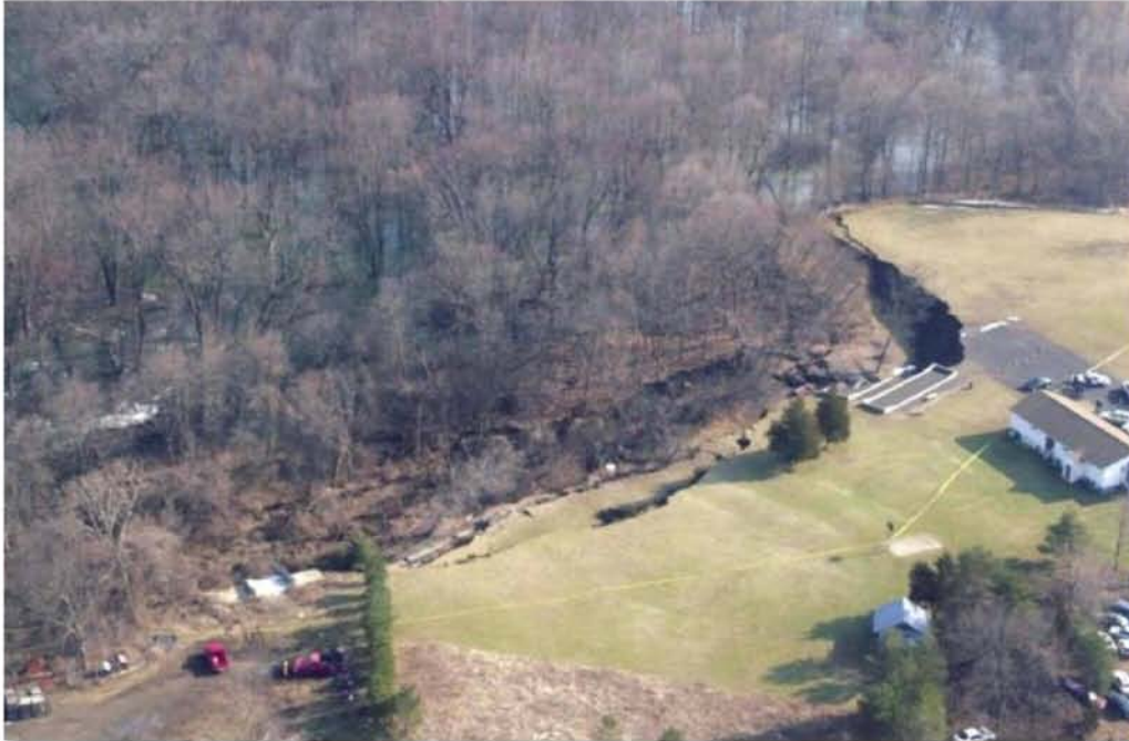
FIG. 1 EROSION, AND ULTIMATELY A SLOPE FAILURE, OF THE OUTSIDE BANK OF A MEANDER
