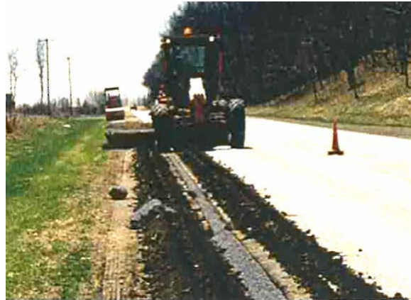
Figure 9-25j PGED: Capping Operation
