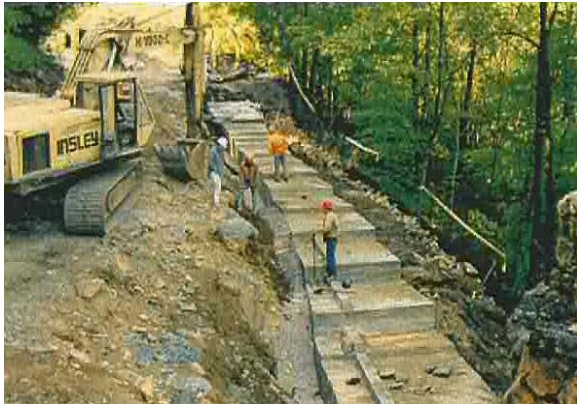
Figure 9-53a Precast Gravity Wall (Foundation Construction)
