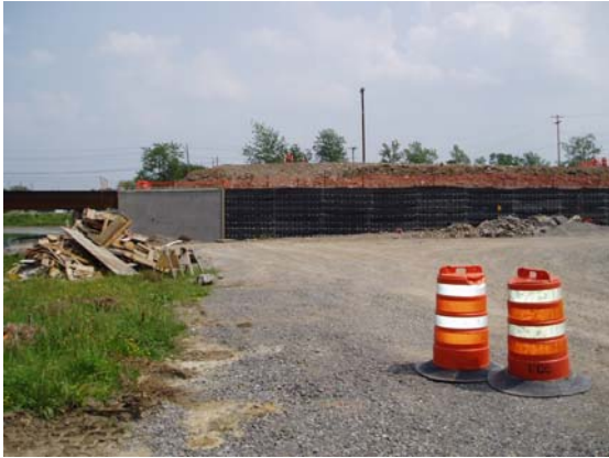
Figure 9-14a Surcharge of Approach Embankment (Additional Fill)
