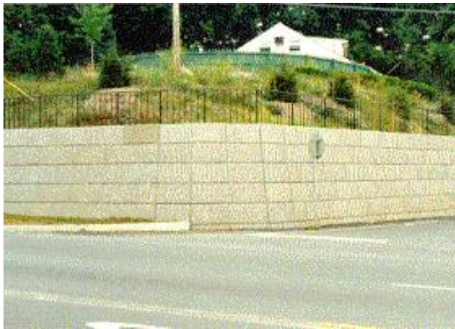
Figure 9-42c Sta-Wall: Exposed Aggregate Finish (Elevation View)
