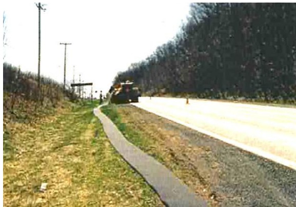
Figure 9-25f PGED: Drain Unrolled
