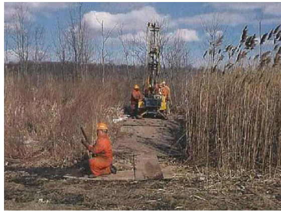
Figure 9-1f Drilling on Soft Soils
