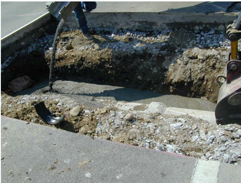
Figure 9-41b Placement of CLSM
