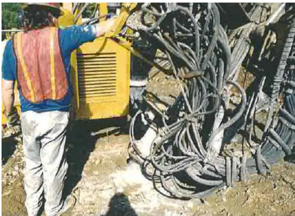
Figure 9-34c Rock Excavation- Drilling
