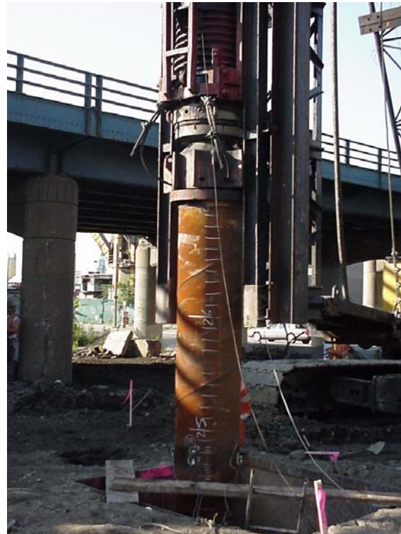
Figure 9-56b Dynamic Pile Load Test Set-Up
