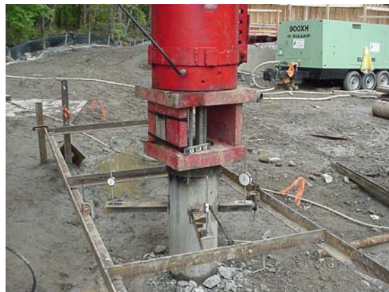
Figure 9-57f Static Pile Load Test of Micropile
