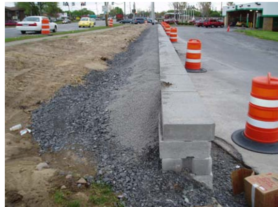
Figure 9-53d Segmental Block Retaining Wall System: Back Face (Unilock Siena Stone 500)
