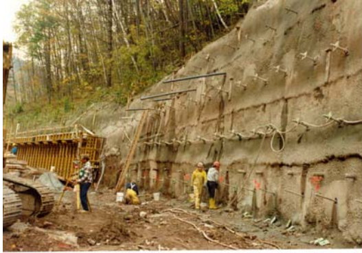
Figure 9-51c Soil Nail Wall (Cast-In-Place Facing)
