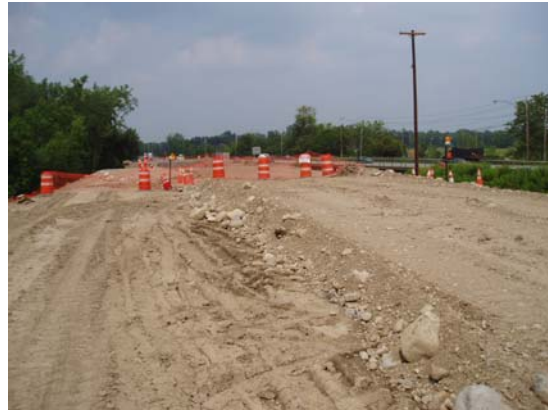
Figure 9-14b Surcharge of Approach Embankment (Instrumentation of Fill)
