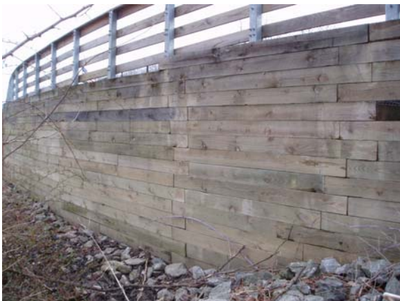
Figure 9-50a Timber Faced GRES Wall
