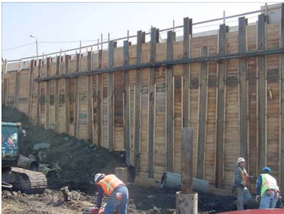
Figure 9-43c Anchored Soldier Pile & Lagging Wall
