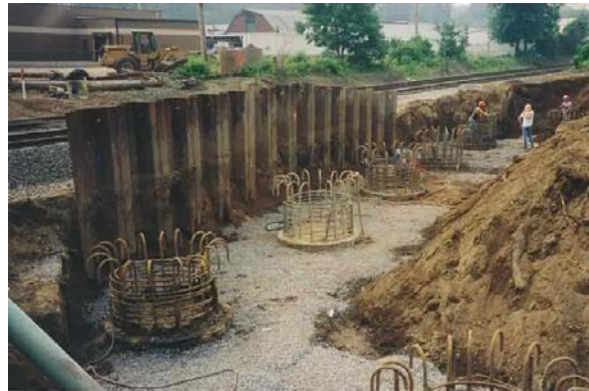
Figure 9-55e Drilled Shaft Layout
