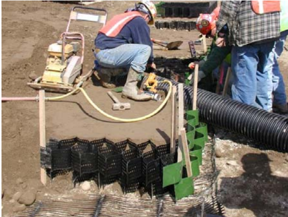
Figure 9-49a Geocell Faced GRES
