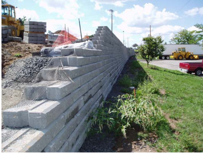
Figure 9-52a Mechanically Stabilized Segmental Block Wall System (Unilock Siena Stone 500 & Strata grid 200)
