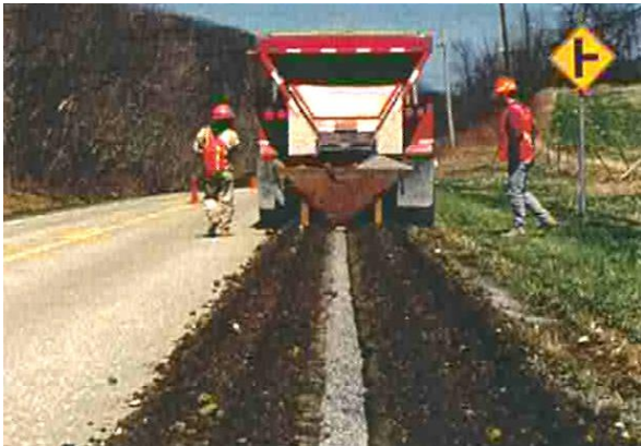
Figure 9-25i PGED: Granular Backfill Material (Pavement/Inner side of trench)
