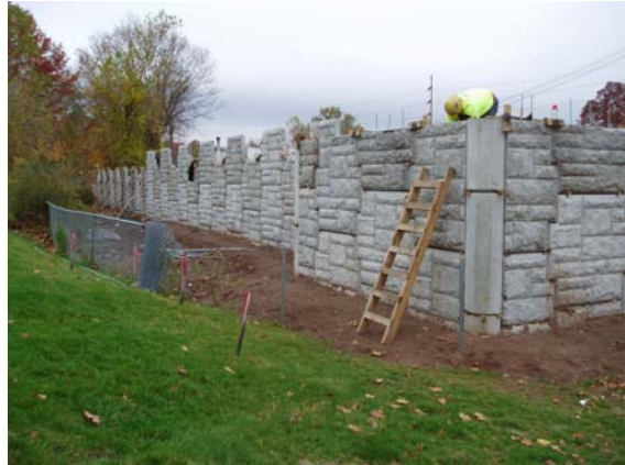
Figure 9-46b MSE Wall (Form Liner Finish)
