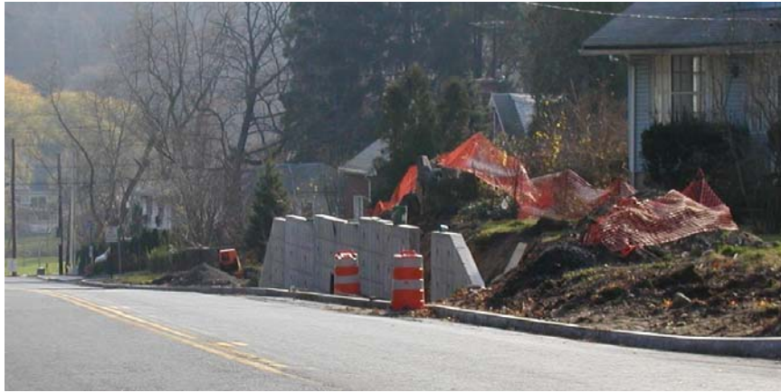
Figure 9-53e Precast Concrete Cantilever Wall
