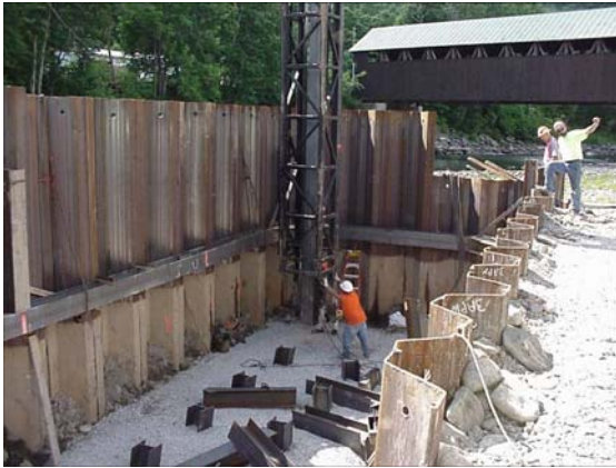
Figure 9-43a Sheeting Wall (Braced Excavation)
