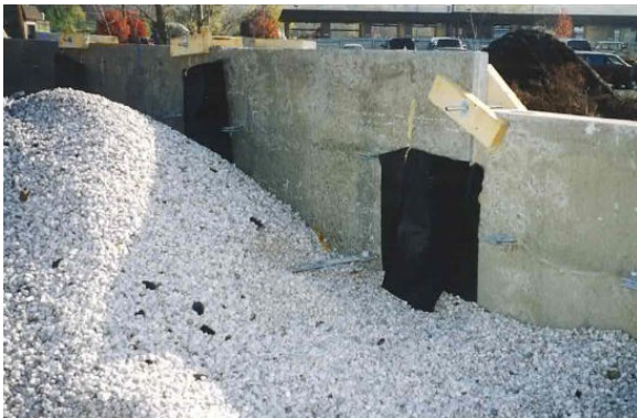
Figure 9-13g Lightweight Fill-Pumice
