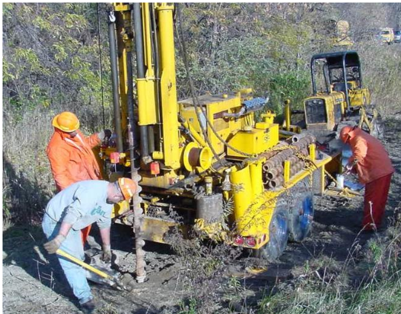
Figure 9-3a Drilling with Augers
