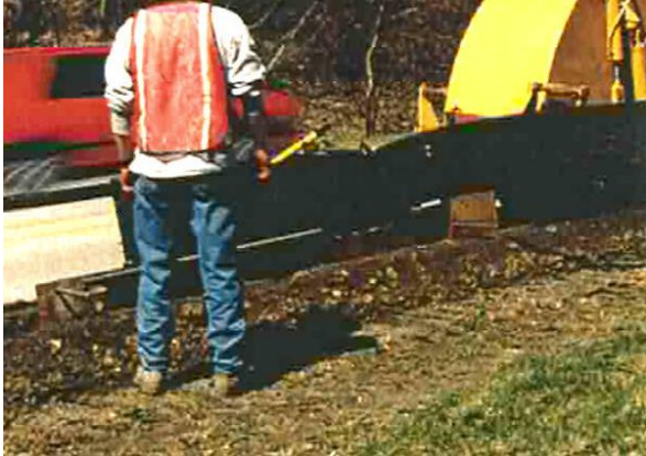
Figure 9-25g PGED: Drain Installed Through Guides
