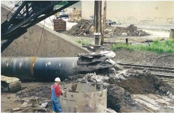
Figure 9-55b Drilled Shaft Installation (Drilling & Excavation)
