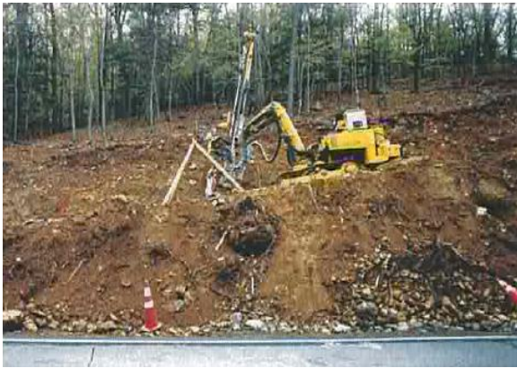
Figure 9-34a Rock Excavation- Drilling
