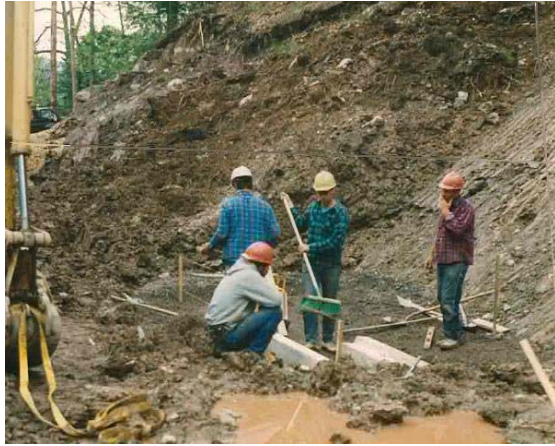
Figure 9-42a Sta-Wall: Plain Concrete Finish (Leveling Beam Installation)
