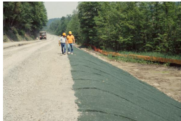
Figure 9-48b GRES (Permanent Oversteepened Slope)
