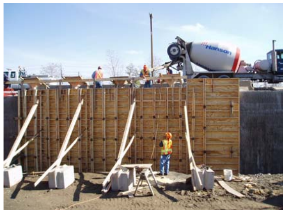
Figure 9-46f MSE Wall (Cast-In-Place Facing)
