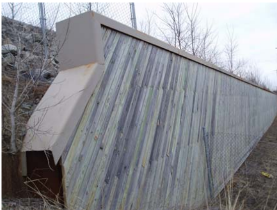
Figure 9-45b Sheeting Wall (Permanent Timber Facing)
