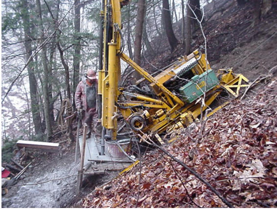
Figure 9-1c Drilling on Steep Terrain
