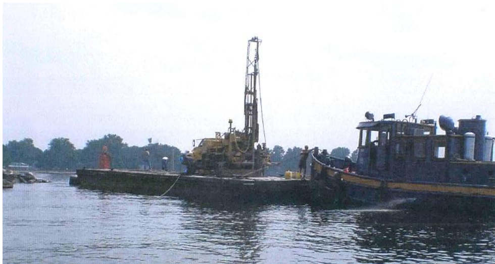
Figure 9-1g Drilling off a Barge
