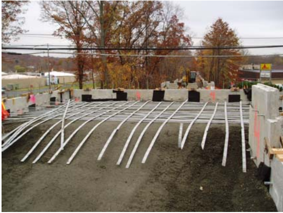
Figure 9-46a MSE Wall (Reinforcement Layout)
