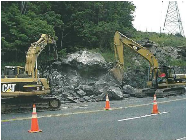
Figure 9-32c Rock Scaling (Using Hoe Ram)
