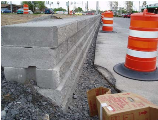
Figure 9-53c Segmental Block Retaining Wall System (Unilock Siena Stone 500)
