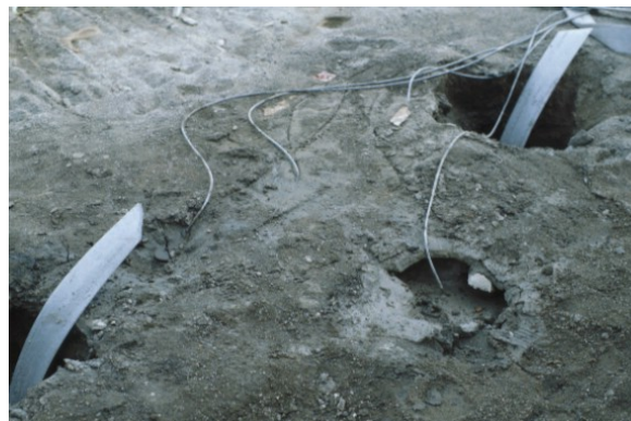
Figure 9-15b Wick Drain Installation (Instrumentation of Some Drains)
