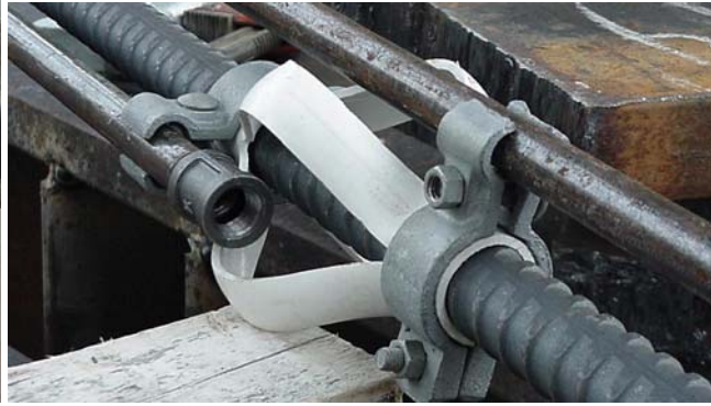
Figure 9-57c Micropile Installation (Centralizer with Telltales)
