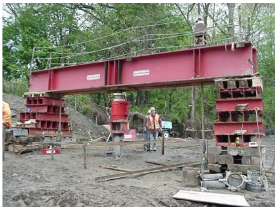
Figure 9-57e Static Pile Load Test of Micropile
