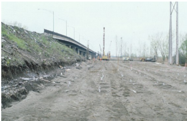
Figure 9-15a Wick Drain Installation (Layout of Drains)
