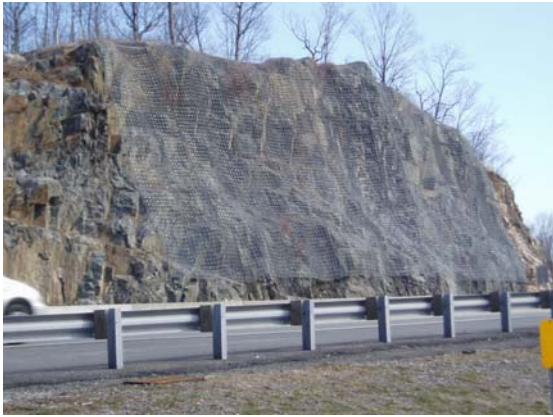
Figure 9-32f Wire Mesh Drape
