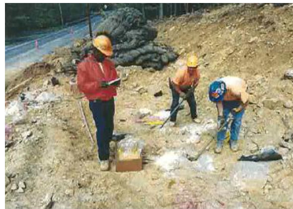
Figure 9-34d Rock Excavation- Explosive Loading
