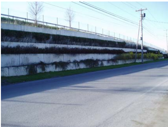
Figure 9-46c Terraced MSE Wall
