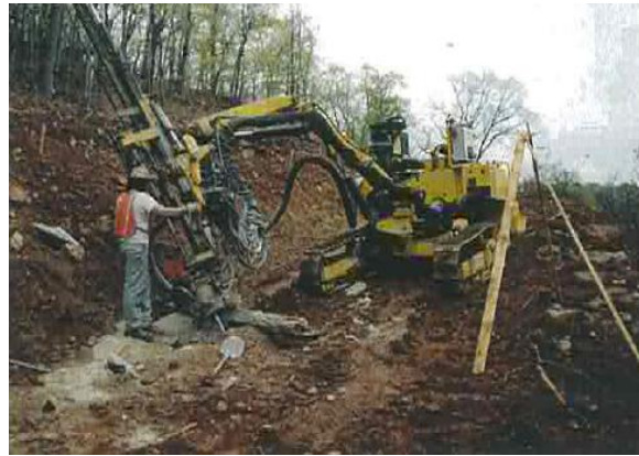
Figure 9-34b Rock Excavation- Drilling
