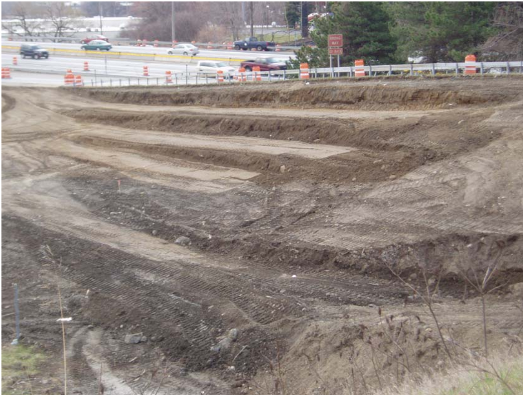
Figure 9-12 Embankment Widening Utilizing Benching
