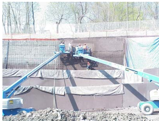
Figure 9-51b Soil Nail Wall (Permanent Shotcrete Facing)
