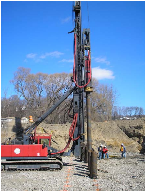
Figure 9-56a Pile Driving Operation
