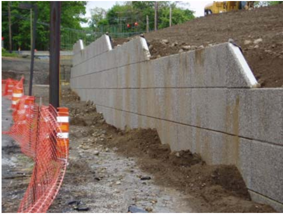
Figure 9-42g T-Wall: Exposed Aggregate Finish (Wall Construction)
