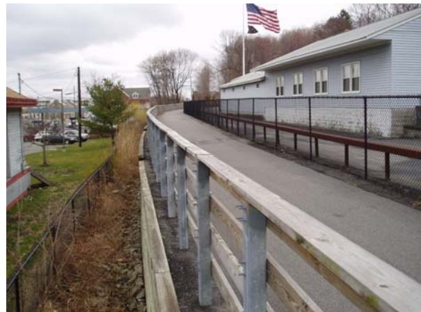
Figure 9-50b Timber Faced GRES Wall
