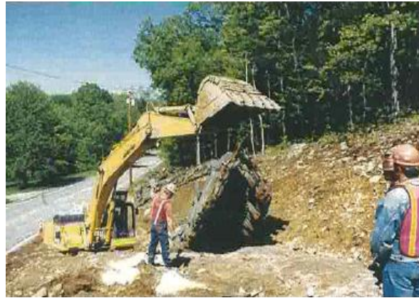
Figure 9-34f Rock Excavation- Matting over Explosives
