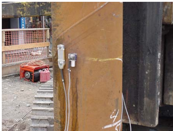
Figure 9-56c DPLT: Strain Transducer and Accelerometer Bolted To CIP Pipe Pile
