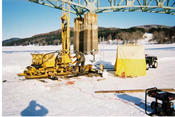
Figure 9-1d Drilling on Ice
