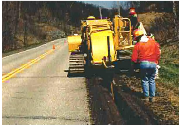
Figure 9-25h PGED: Drain Installed (Outer side of Trench)
