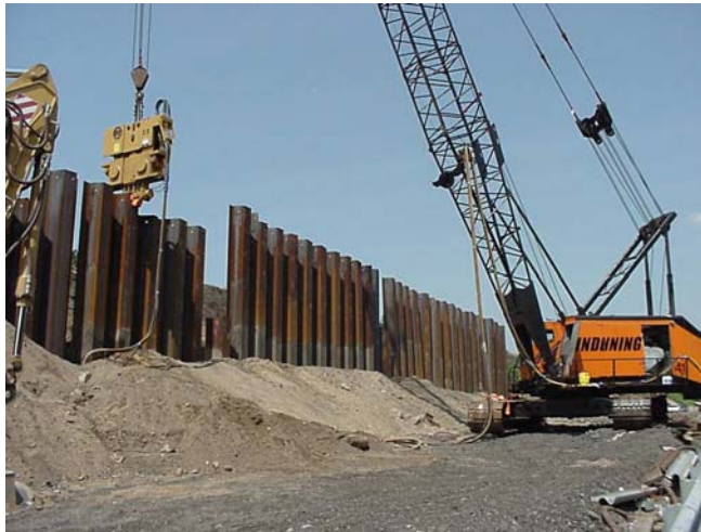
Figure 9-45a Sheeting Wall Installation
