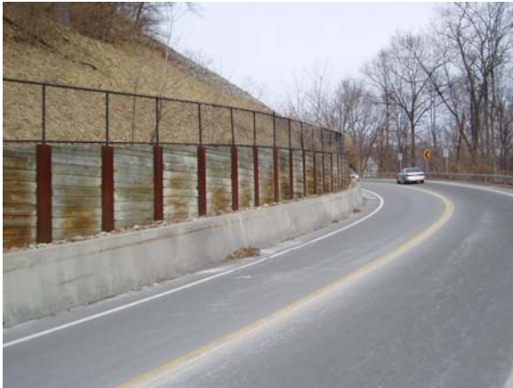
Figure 9-44a Soldier Pile & Lagging Wall (Permanent Timber Lagging)
