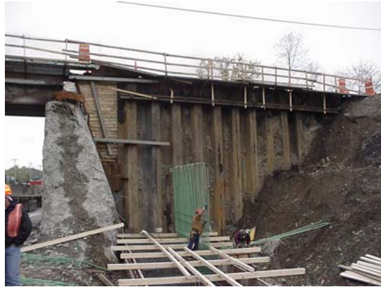
Figure 9-43b Anchored Sheeting Wall
