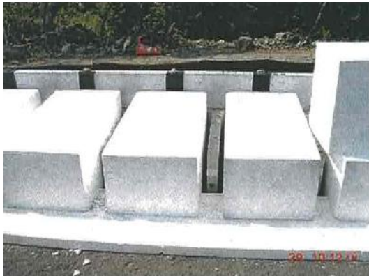
Figure 9-13a Lightweight Fill- Expanded Polystyrene Blocks (EPS)
