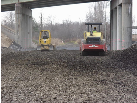
Figure 9-13e Lightweight Fill-Tire Shreds
