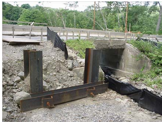
Figure 9-43f Anchor (Soldier Pile Deadman)
