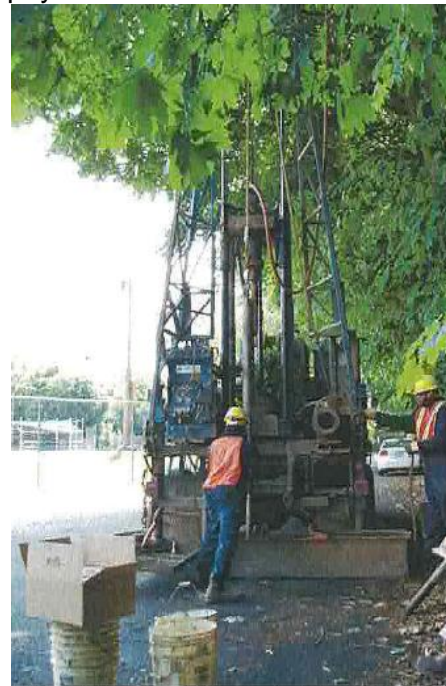
Figure 9-1b Drilling in a Parking Lot
