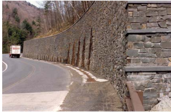
Figure 9-51d Soil Nail Wall (Stone Masonry Facing)
