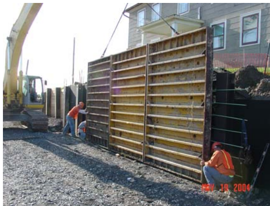
Figure 9-44c Soldier Pile & Lagging Wall (Cast-In-Place Finish)
