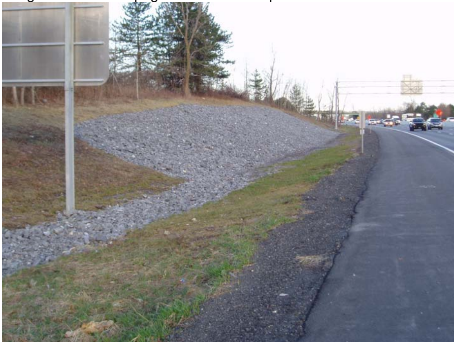
Figure 9-29 Stone Slope Protection
