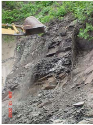
Figure 9-32a Rock Scaling (Using Long Reach Excavator)
