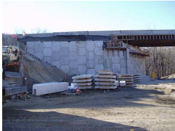
Figure 9-46d MSE Wall (Temporary Stage Line Wall)
