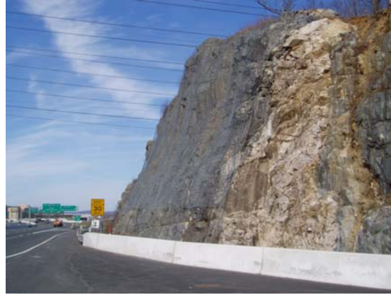
Figure 9-32g Wire Mesh Drape
