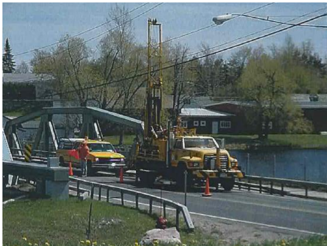
Figure 9-1a Drilling in Roadway
