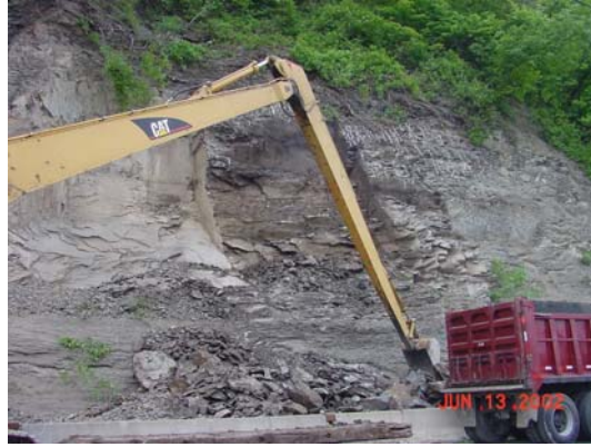
Figure 9-32b Rock Scaling (Using Long Reach Excavator)
