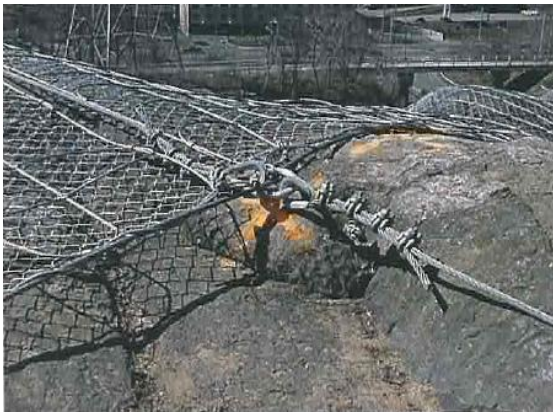
Figure 9-32h Wire Mesh Drape (Drape Connections)
