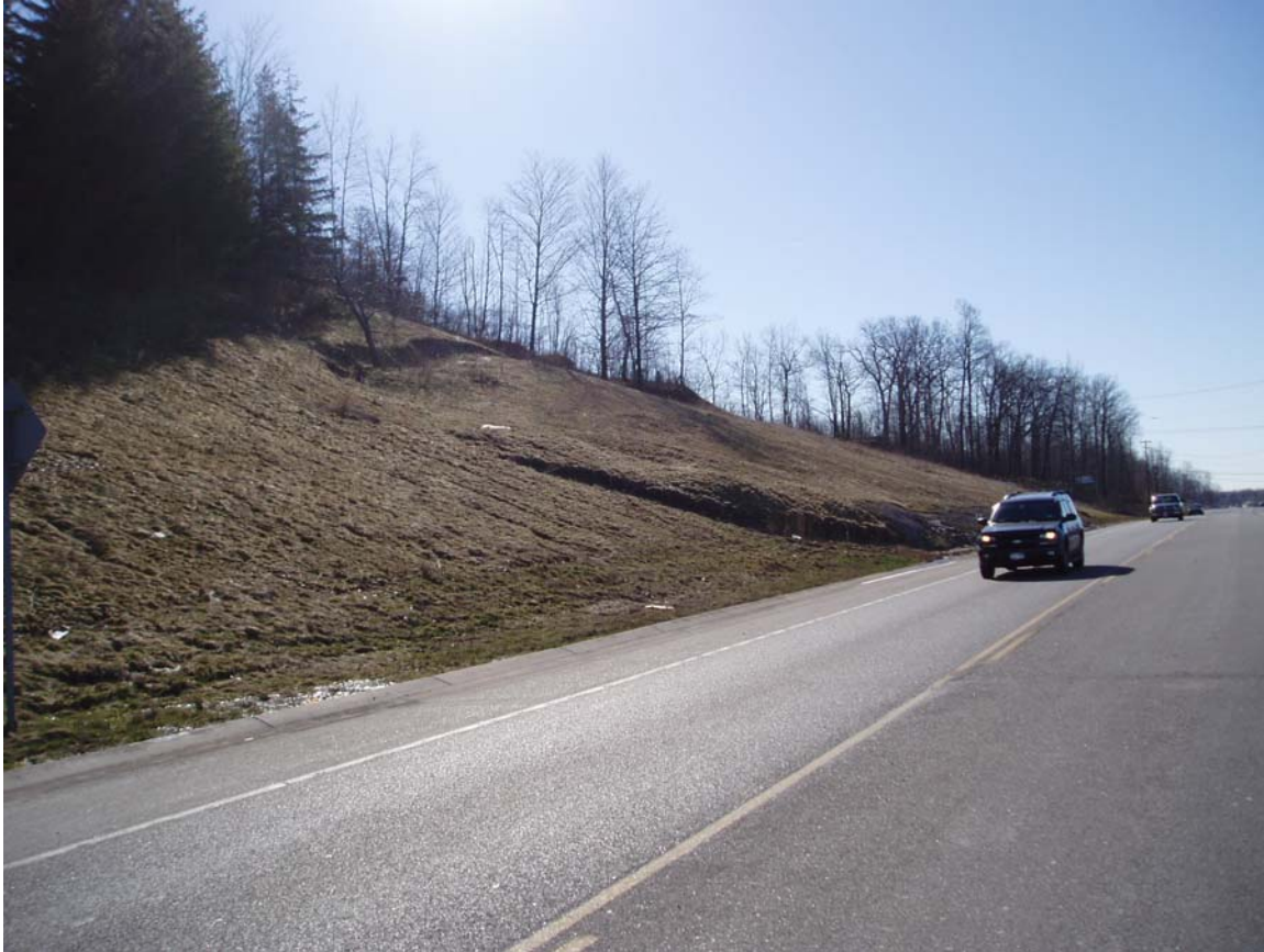
Figure 9-26 Large Scale Surface Slough
