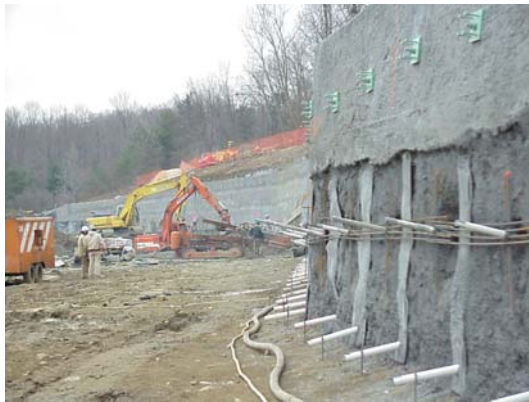
Figure 9-51a Soil Nail Wall (Temporary Shotcrete Facing)
