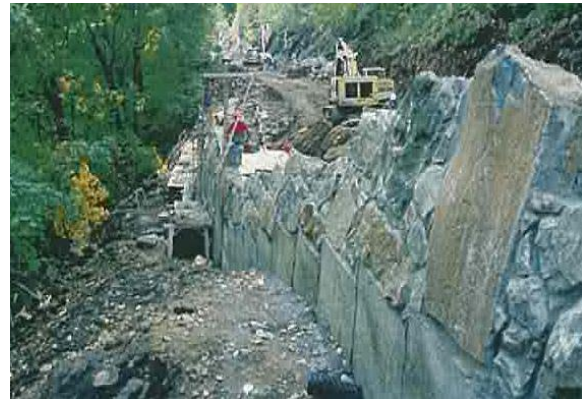
Figure 9-53b Precast Gravity Wall (Stone Facing)
