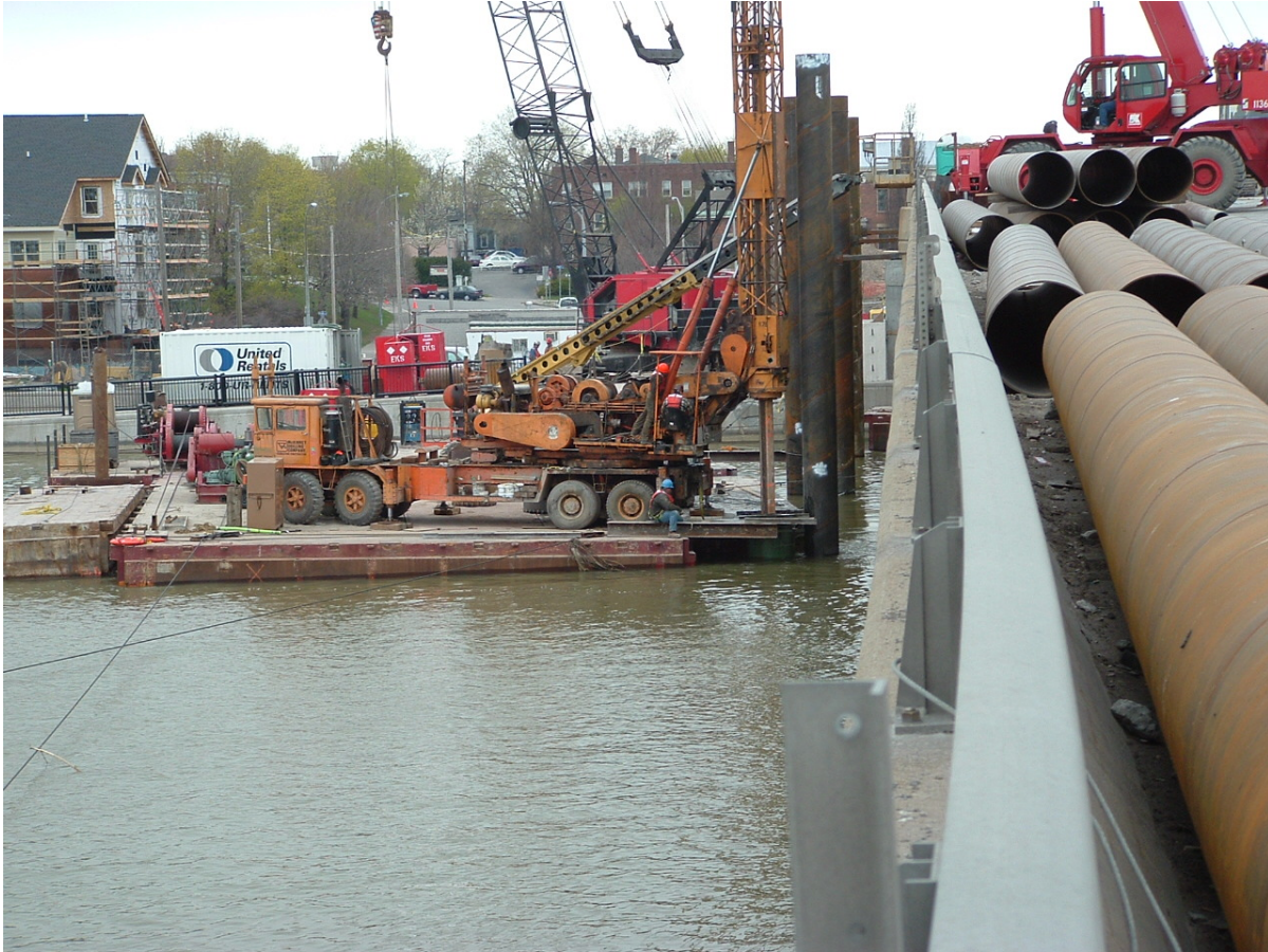
Figure 9-55a Drilled Shaft Installation (Barge Set-Up)
