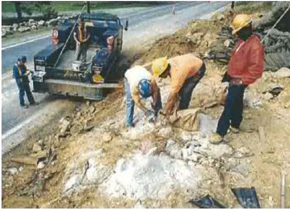
Figure 9-34e Rock Excavation- Explosive Loading
