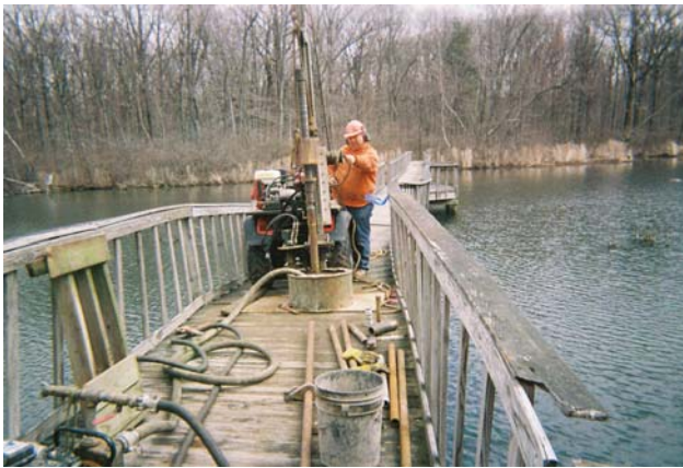
Figure 9-1e Drilling with an All-Terrain Vehicle (ATV) Drill Rig
