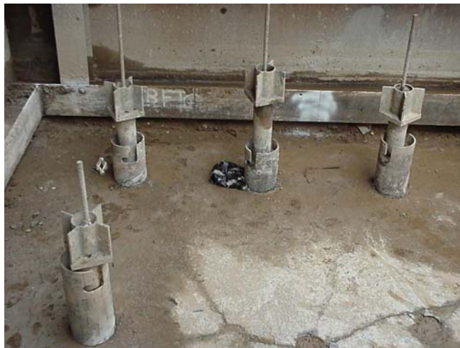
Figure 9-57d Micropile Installation (Footing Connection)
