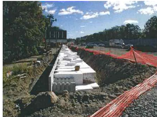
Figure 9-13b Lightweight Fill- Expanded Polystyrene Blocks (EPS)
