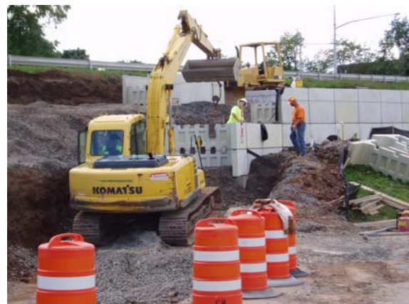
Figure 9-42f T-Wall: Plain Concrete Finish (Wall Construction)
