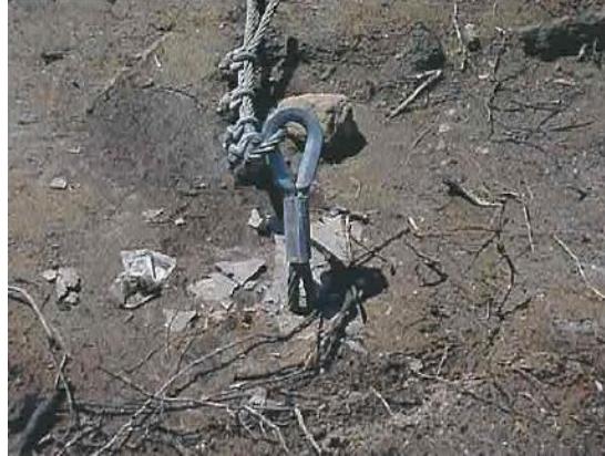
Figure 9-32i Wire Mesh Drape (Anchor)
