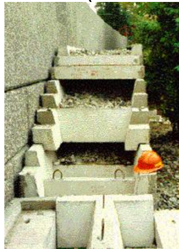
Figure 9-42d Sta-Wall: Exposed Aggregate Finish (Stair Construction)
