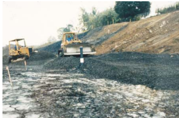
Figure 9-13j Lightweight Fill-Expanded Shale
