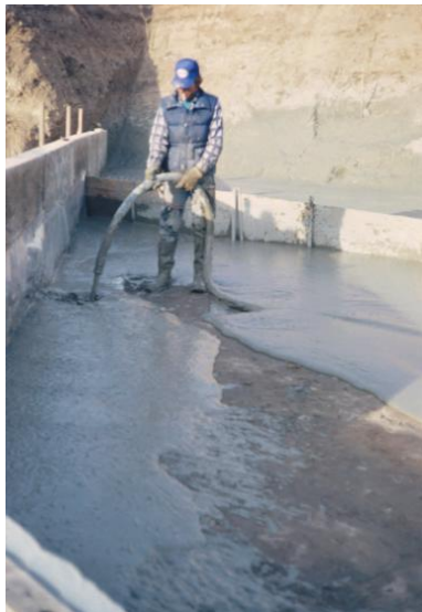
Figure 9-13c Lightweight Foamed Concrete
