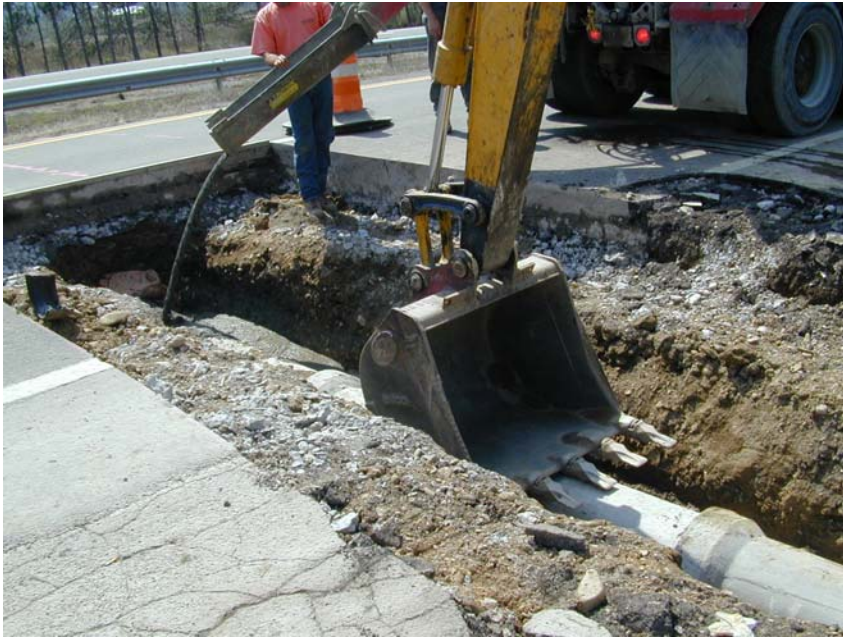
Figure 9-41a Placement of CLSM
