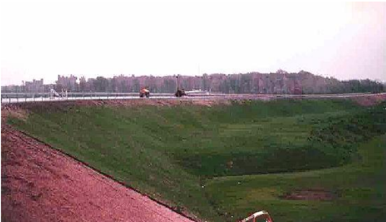
Figure 9-20 Constructed Stabilization Berm
