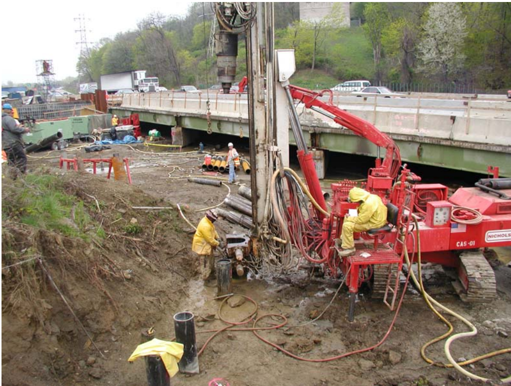
Figure 9-57a Micropile Installation
