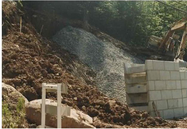
Figure 9-42b Sta-Wall: Plain Concrete Finish (Wall Construction)
