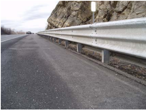
Figure 9-32l Thrie Beam Railing/ Corrugated Beam Rock Fence
