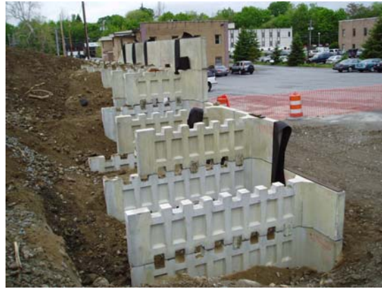
Figure 9-42h T-Wall: Exposed Aggregate Finish (Wall Construction)
