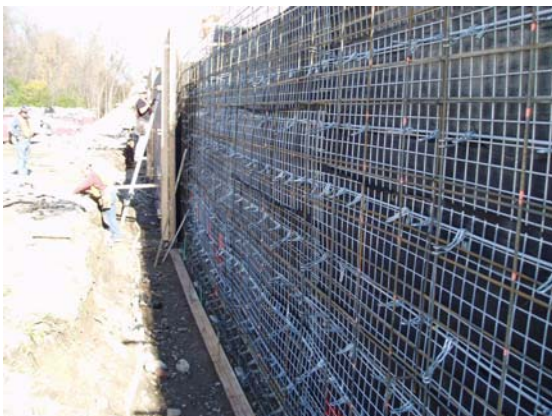
Figure 9-46e MSE Wall (Cast-In-Place Facing)
