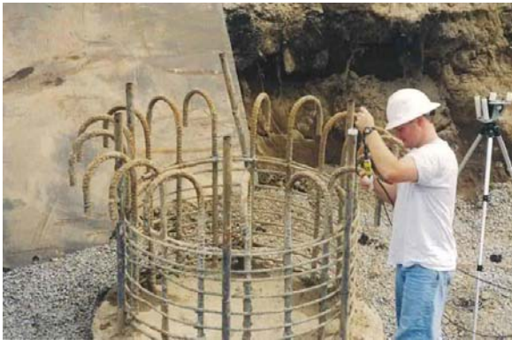
Figure 9-55f Crosshole Sonic Log Testing (Ultrasonic Probe Installation)
