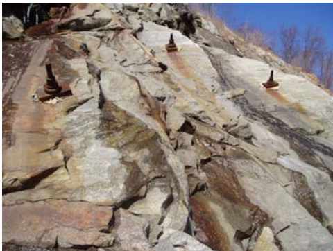
Figure 9-32d Rock Bolts
