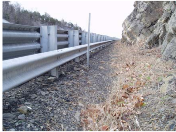
Figure 9-32m Thrie Beam Railing/ Corrugated Beam Rock Fence
