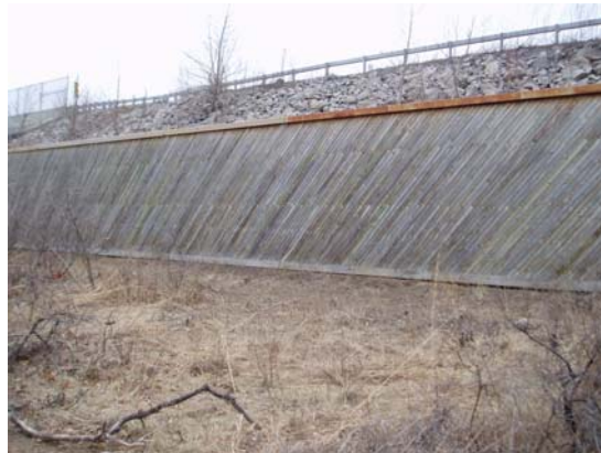
Figure 9-45c Sheeting Wall (Permanent Timber Facing)
