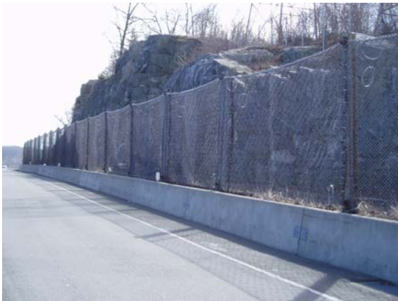
Figure 9-32n Wire Rope Catchment Fence (Medium Impact)
