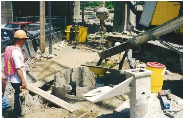
Figure 9-55d Drilled Shaft Installation (Concrete Pour)
