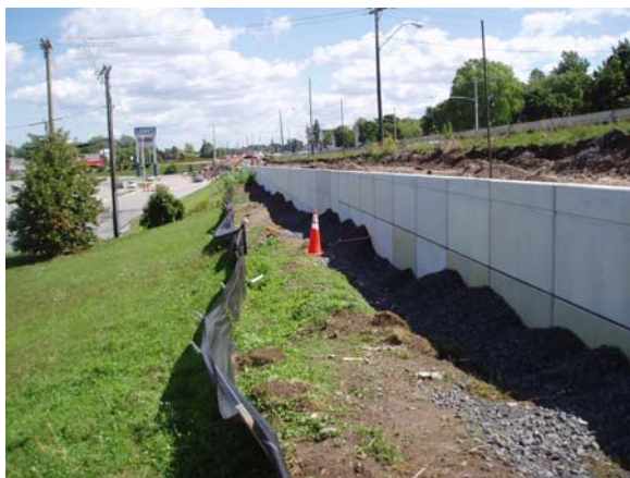
Figure 9-42e T-Wall: Plain Concrete Finish (Wall Construction)
