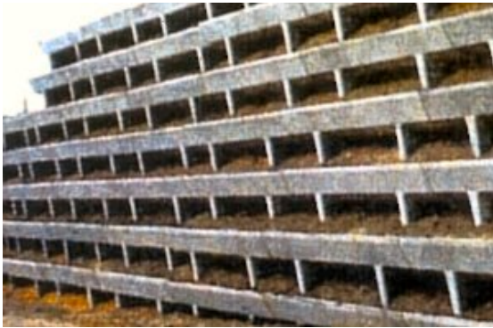
Figure 9-42i Evergreen Wall (Constructed Wall)
