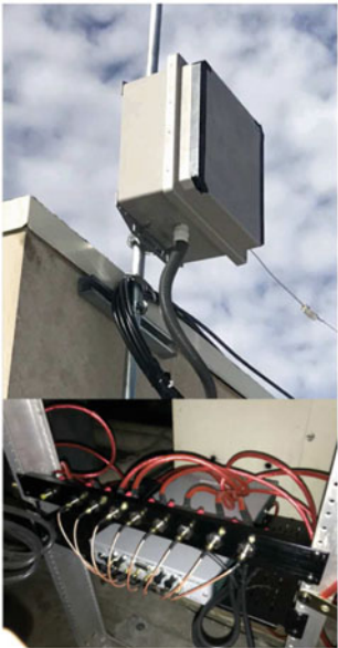
(b) Rooftop Antenna & Transceiver Mounting
