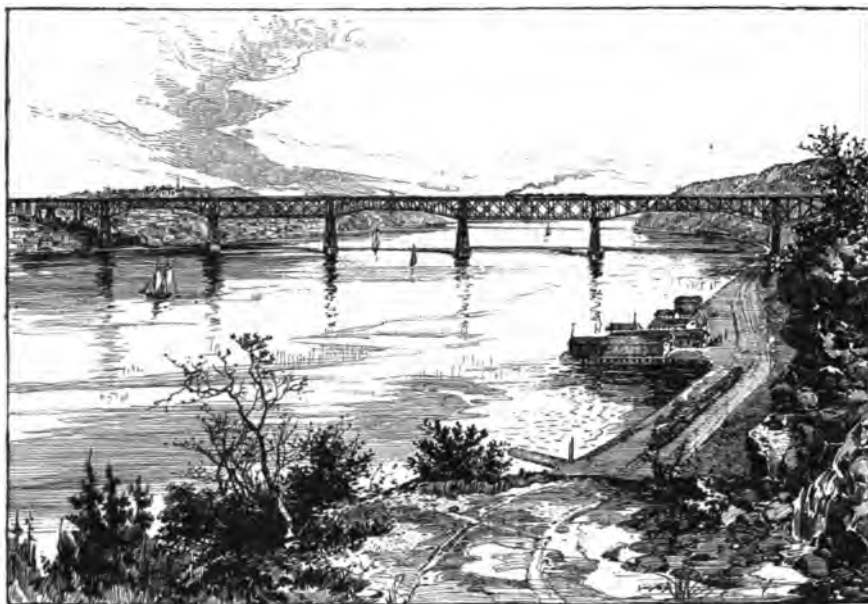
General View of the Poughkeepsie Bridge.
