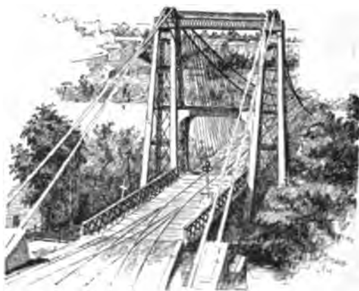
The New Iron Towers of the Same.
