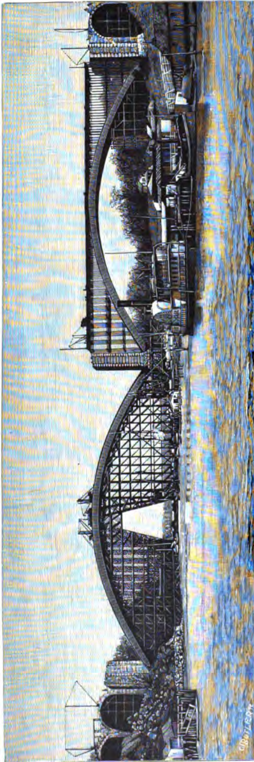
The 510-foot Span Steel Arches of the New Harlem River Bridge, New York, during construction.
