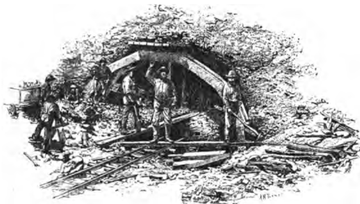
Beginning a Tunnel.
