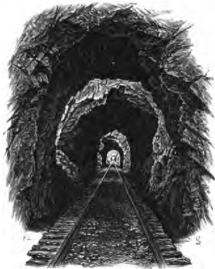
A Series of Tunnels.
