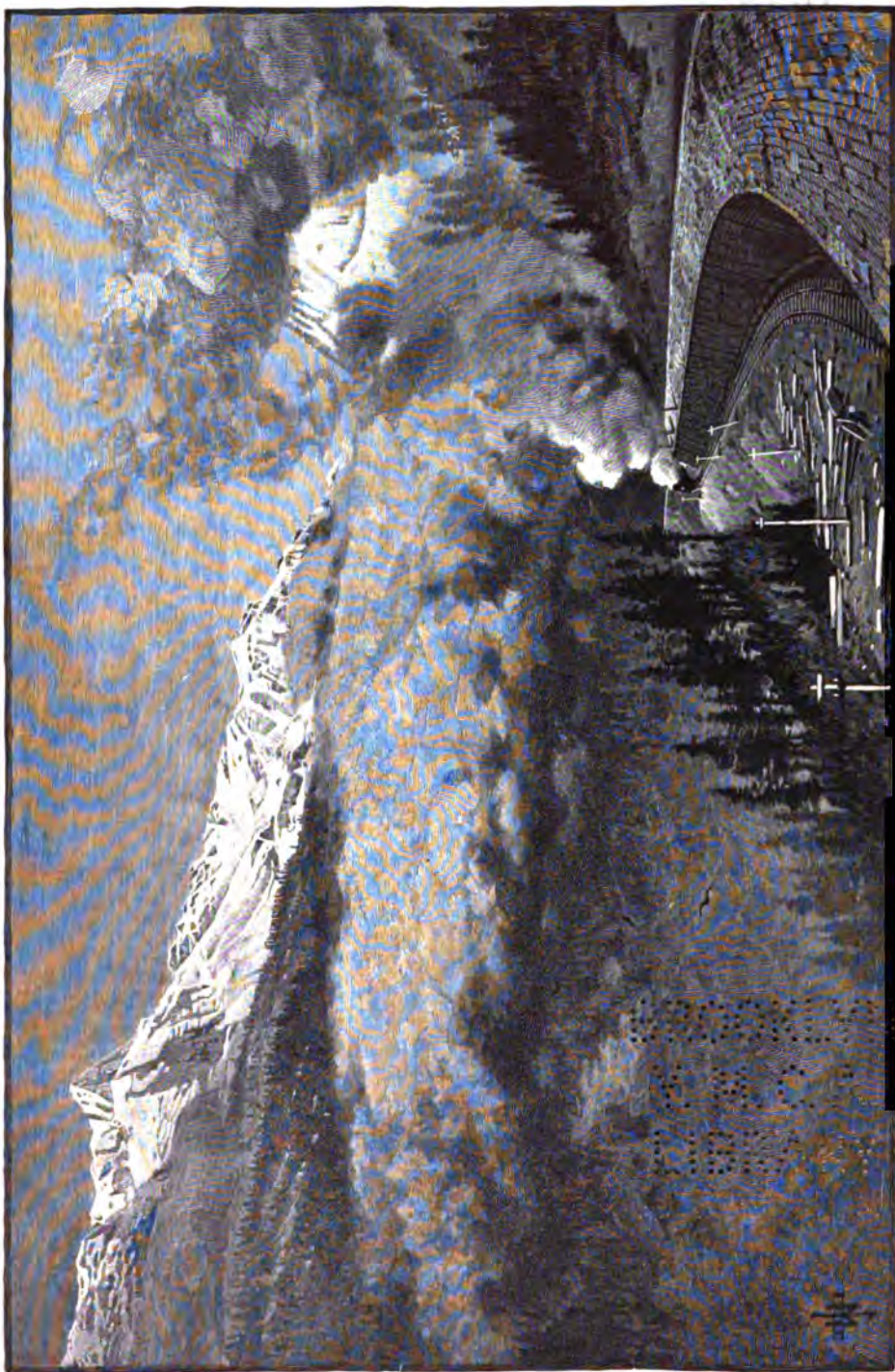
Snow-sheds, Selkirk Mountains, Canadian Pacific. The winter track under cover; the outer track for summer use.
